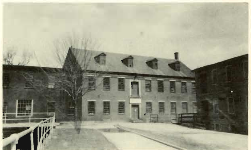
Machine Shop - Building #10
