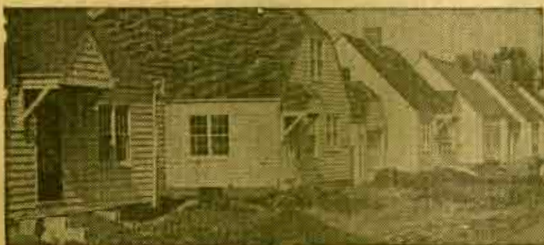
Row on row of pretty little cottages will be built, provided building costs are kept at levels that can be reached by the majority of prospective purchasers.
